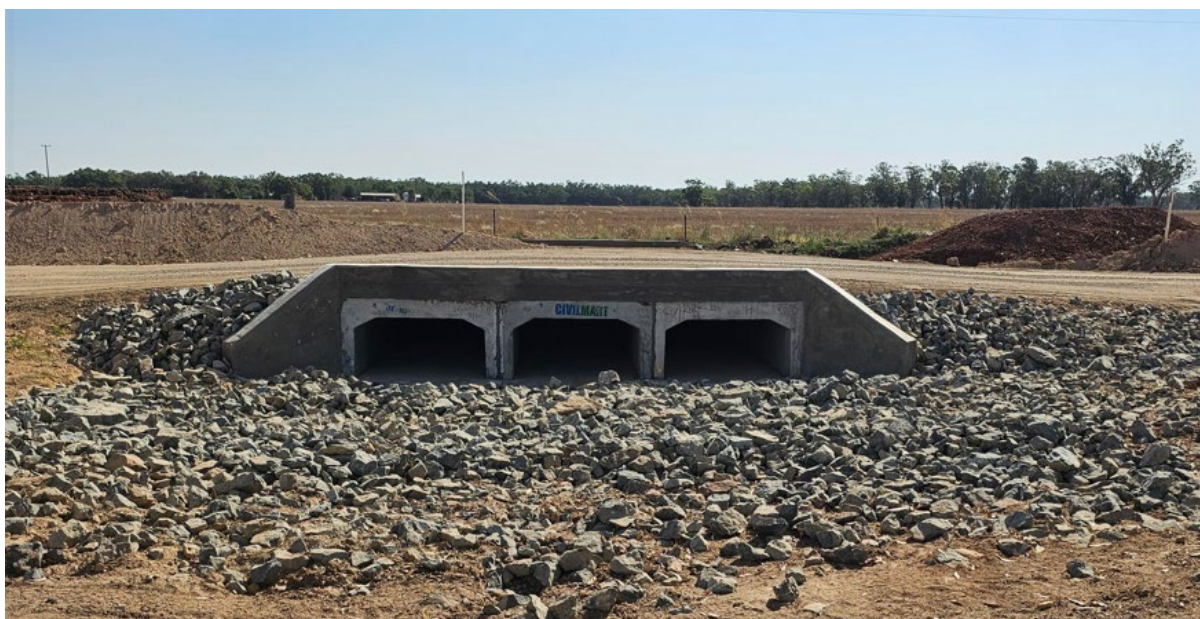
Figure 3: New Culvert on Frecklingtons Crossing
