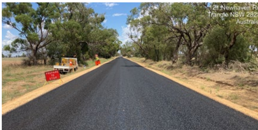
Figure 2: Newhaven Road has been upgraded and sealed
