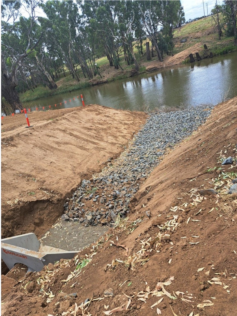
Figure 8: The northern drainage river outlet has been constructed
